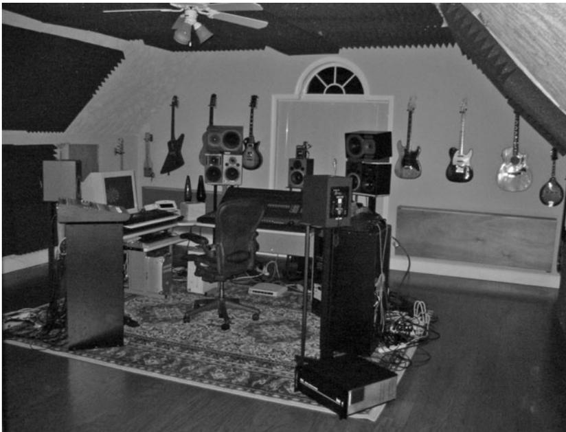
**Figure R.3** A Reflection-Free Zone is an area in a control room where all reflections have been controlled, increasing the accuracy of monitoring. In this case, absorptive acoustic foam has been mounted around the listening position to control reflections.
